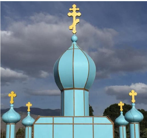
Renovation of Dome Completed
