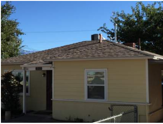
New roof for the rectory
