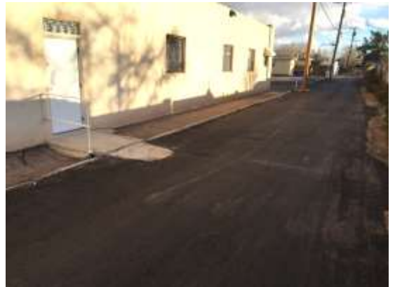
New Asphalt on the back alley
